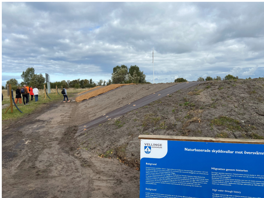
Figure 3. A full-scale model of the dikes that will be built on the Falsterbo peninsula to protect the settlements, with information board on “Nature-based dikes against flooding”. Photograph: Carola Wingren. Used by kind permission.
